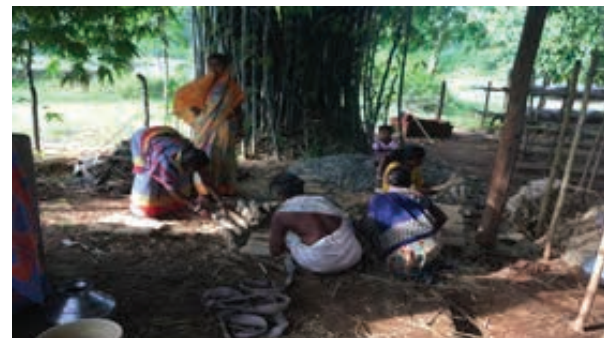
Preparation for laying bed
