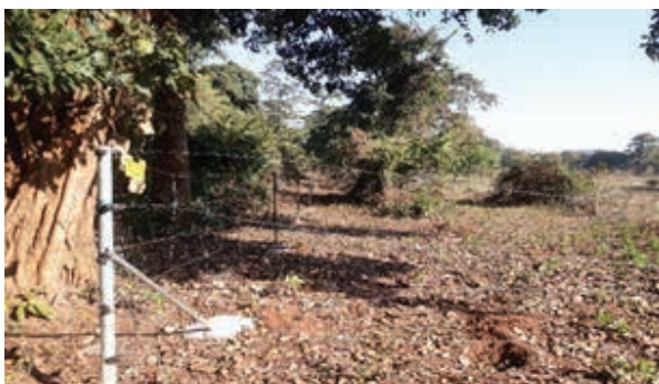
Photo-voltaic (solar) fencing, Nunvet
