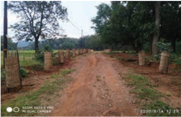
Plantation work completed, Badi Bahal
