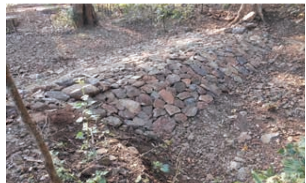
The Nalas Treated with LBDC structures, Nunvet
